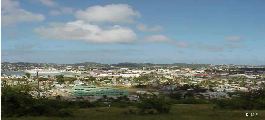
Photograph 1: Overview of St. John's
